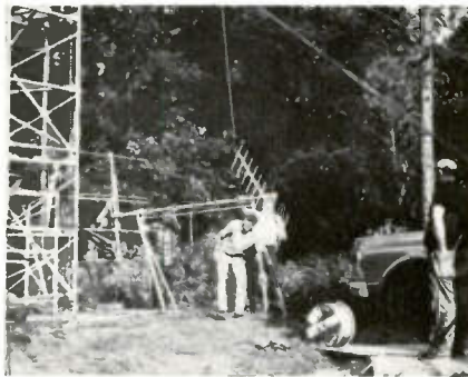
Fifteen man crew assembling 300 ft. tower.
