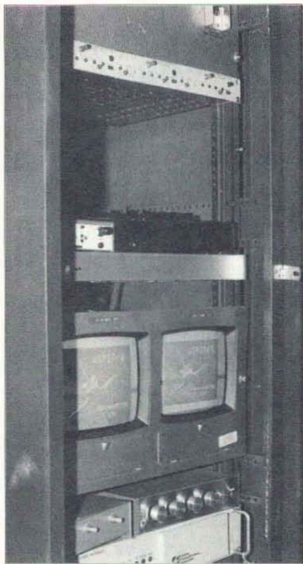
Photo B. Monitors and controllers at the HATS ATV repeater transmitter site.
