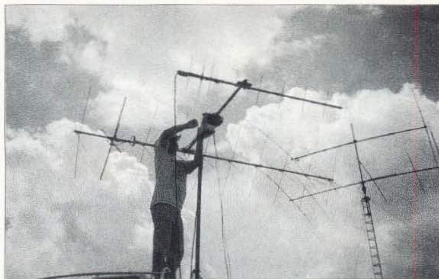
Photo C. Mike WA5TWT finishes installation of the VHF/UHF array at one of the K5DX hamsat stations.
