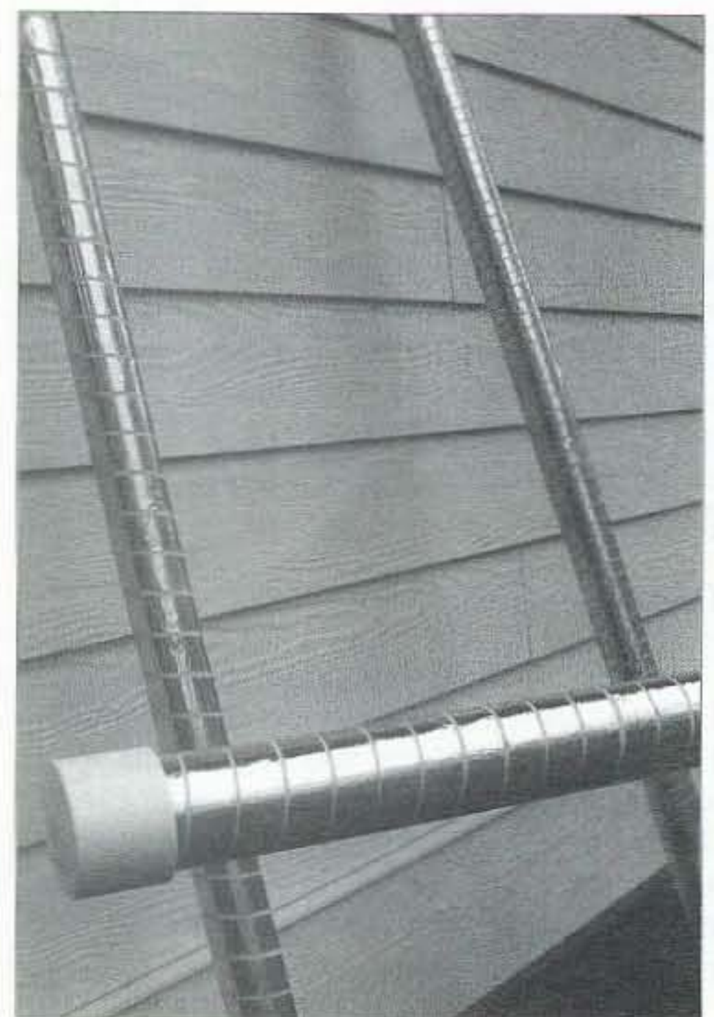
Photo B. Here's how to wind the tape onto the mast: close, but not touching.
