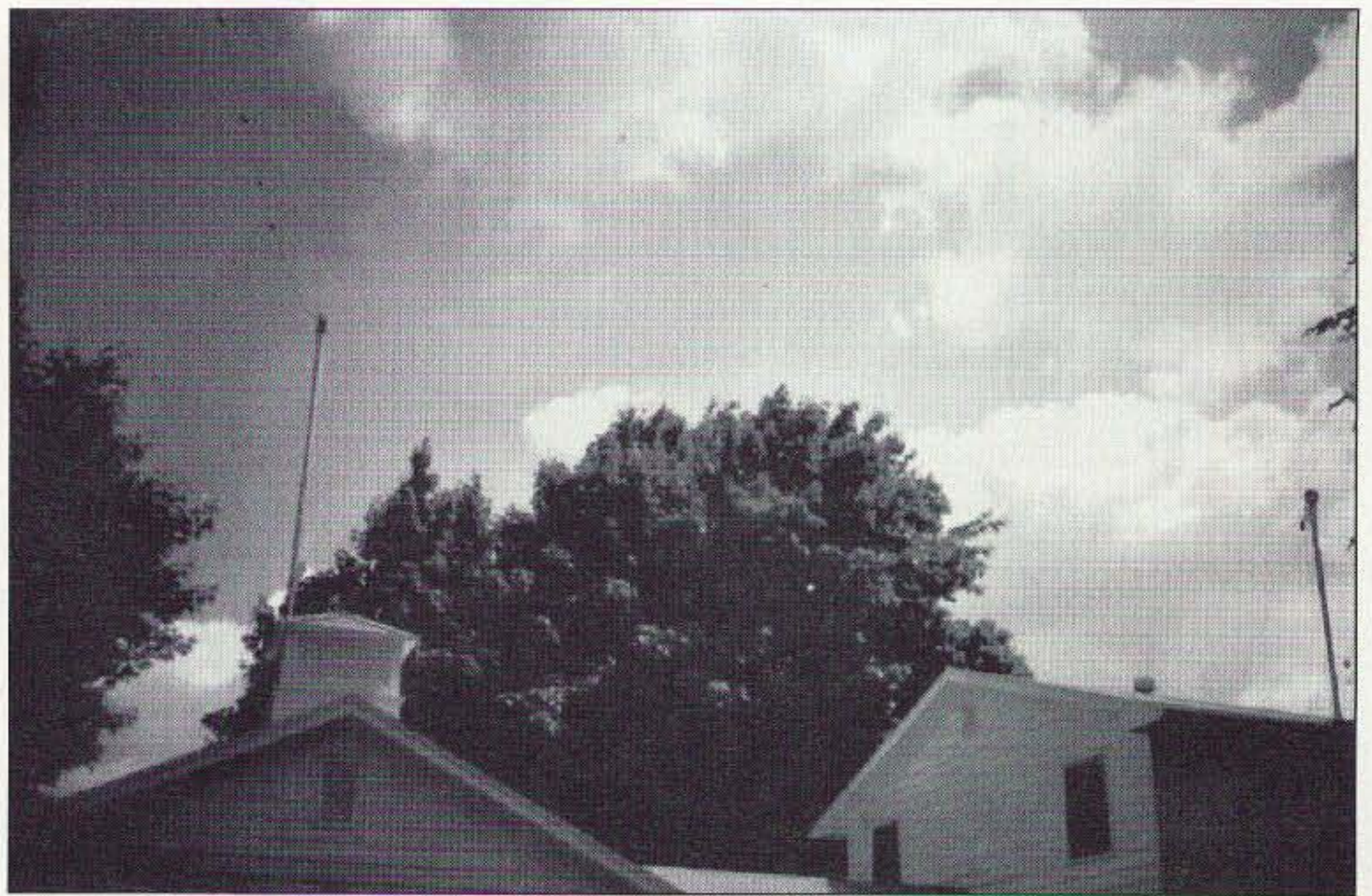
Photo C. The radiator, suspended by two 40-foot-high masts. The box is at the lefthand mast and the center insulator is near the righthand mast.
