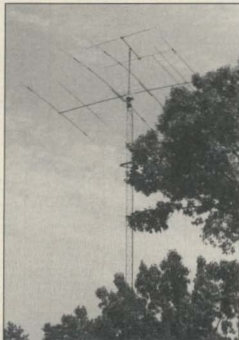
Photo E. The installed Pro-67, ready for action. [Photo by author.]
