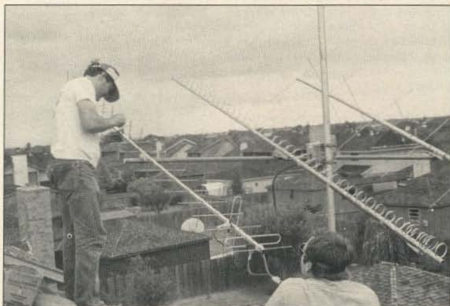
Photo C. WA5ZIB and WA5WOD fine tune element alignment on the 70 cm antenna.
