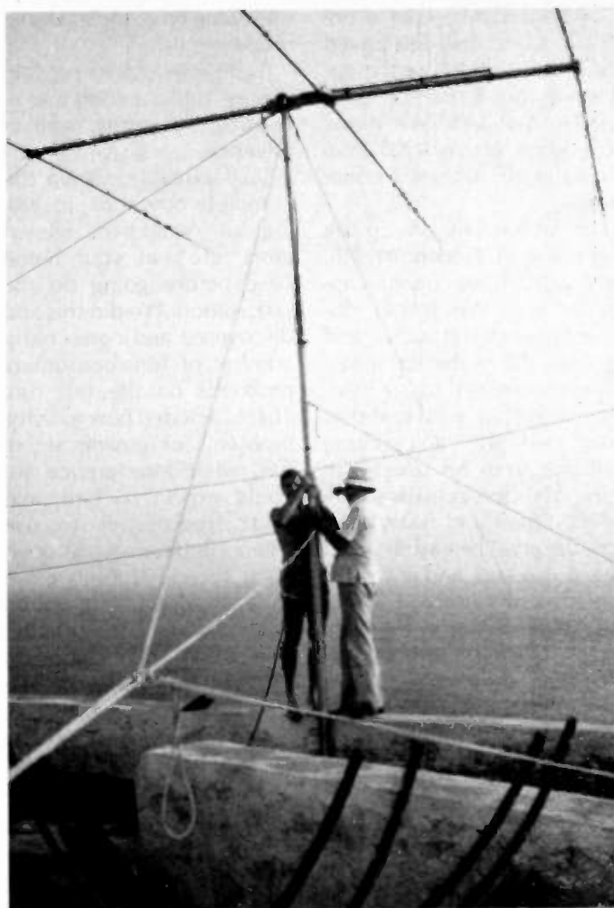
Jean F6GBQ (left) and Lloyd W6KC erecting an antenna on Abu Ail. It is 350' almost straight down to water behind them.
