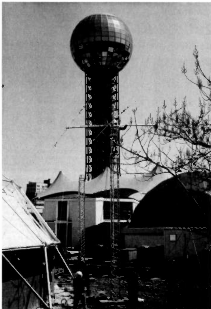
While the health pavilion was being finished, local hams installed two towers, tribanders, a 2-meter antenna, and dipoles.
