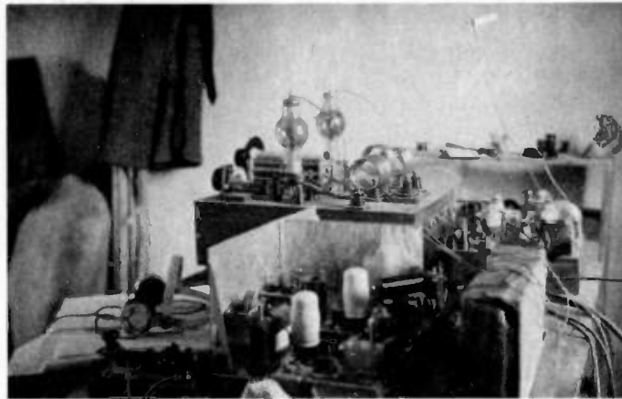
The transmitter, receiver, and Collins coupler installed in the barracks at Gyantse.
