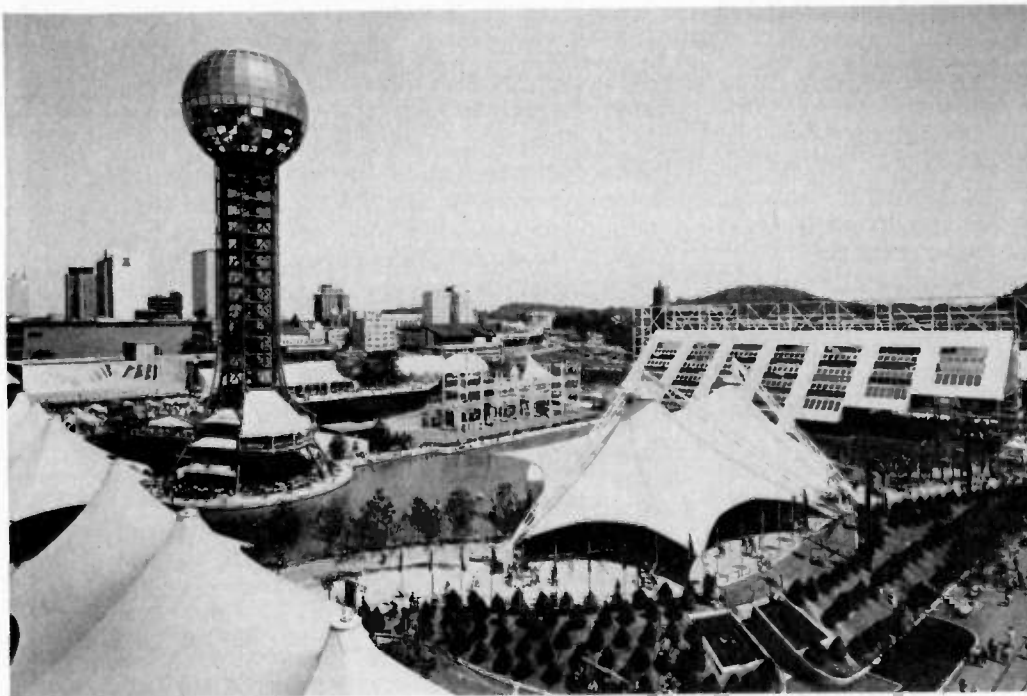
Three of the landmark structures of The 1982 World's Fair in Knoxville, Tennessee, form around the three-acre Waters of the World Lake. At left is the Sunsphere, 266 feet high and the "theme structure" of the exposition. The five-level sphere, encased in glass made of 24-karat gold dust, houses a restaurant and two cocktail lounges and observation areas. In the right foreground is the 1,500-seat Tennessee State Amphitheatre. The United States pavilion (at far right) features "talk-back computers," a "national energy debate" utilizing television screens and a new IMAX film, to be shown on a screen seven stories high and 90 feet wide. Downtown Knoxville forms the background at left. (Photo by Mike DuBose)
