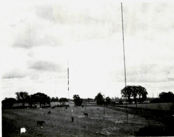
Photo B. Transmitting antennas.
