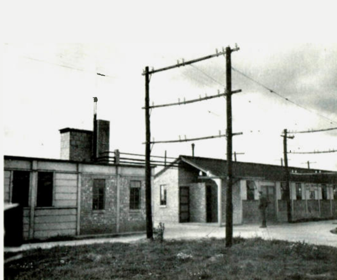
Photo D. Transmitter Building.
