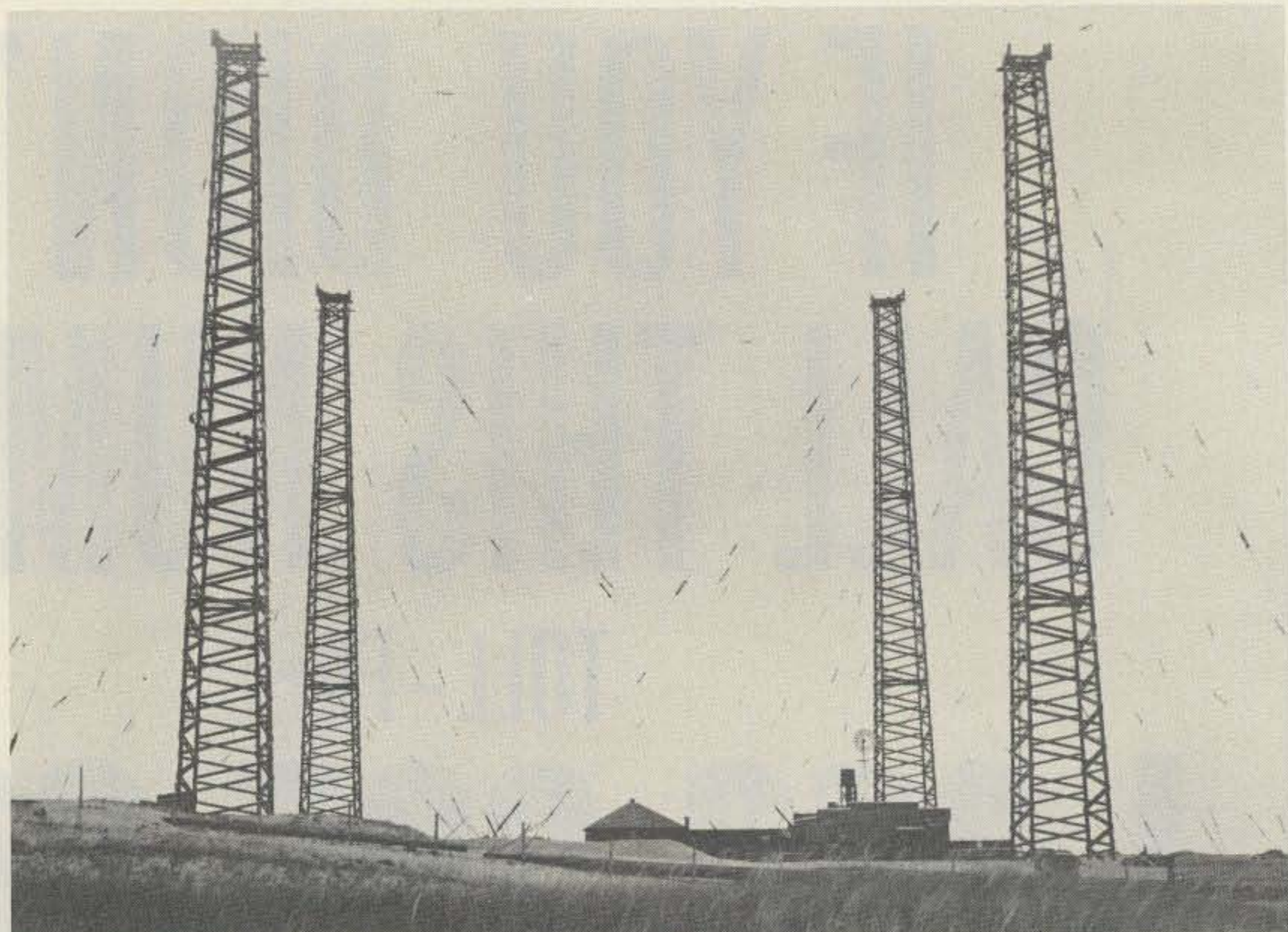
Photo B. These Cape Cod towers were made of wooden planks similar to those described in the text. Close inspection reveals a man about halfway up the tower on the far left (look for him on the left edge of the tower).
