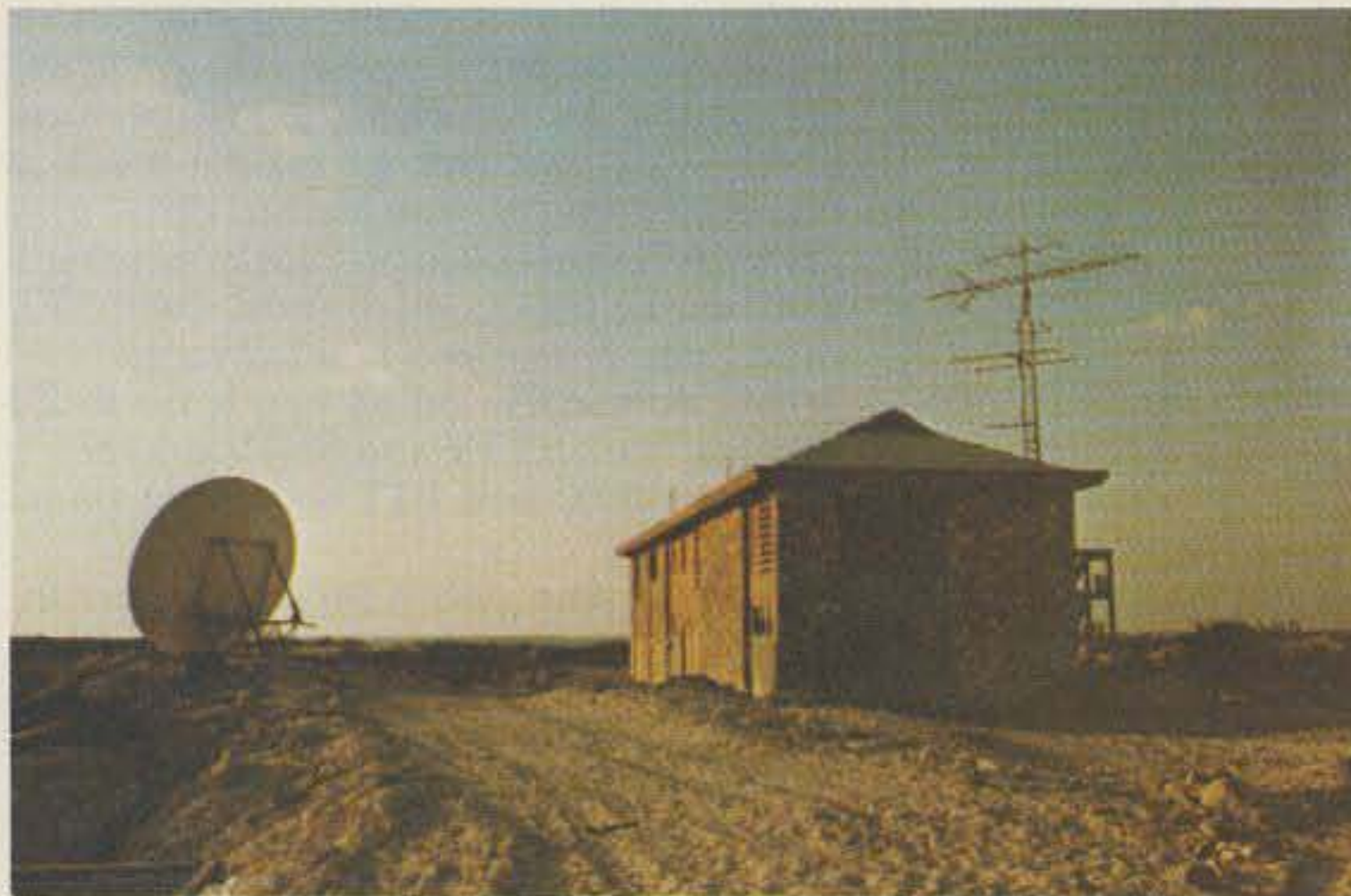
The dish and studio building of WIV. The antennas pick up TV from Miami during openings. They also send the satellite signals via channel 7 to a hilltop, where a solar-powered transmitter rebroadcasts on channel 4 for the whole island. It's free for now, but Bob intends to encode the signals and charge . . . much like cable TV.
