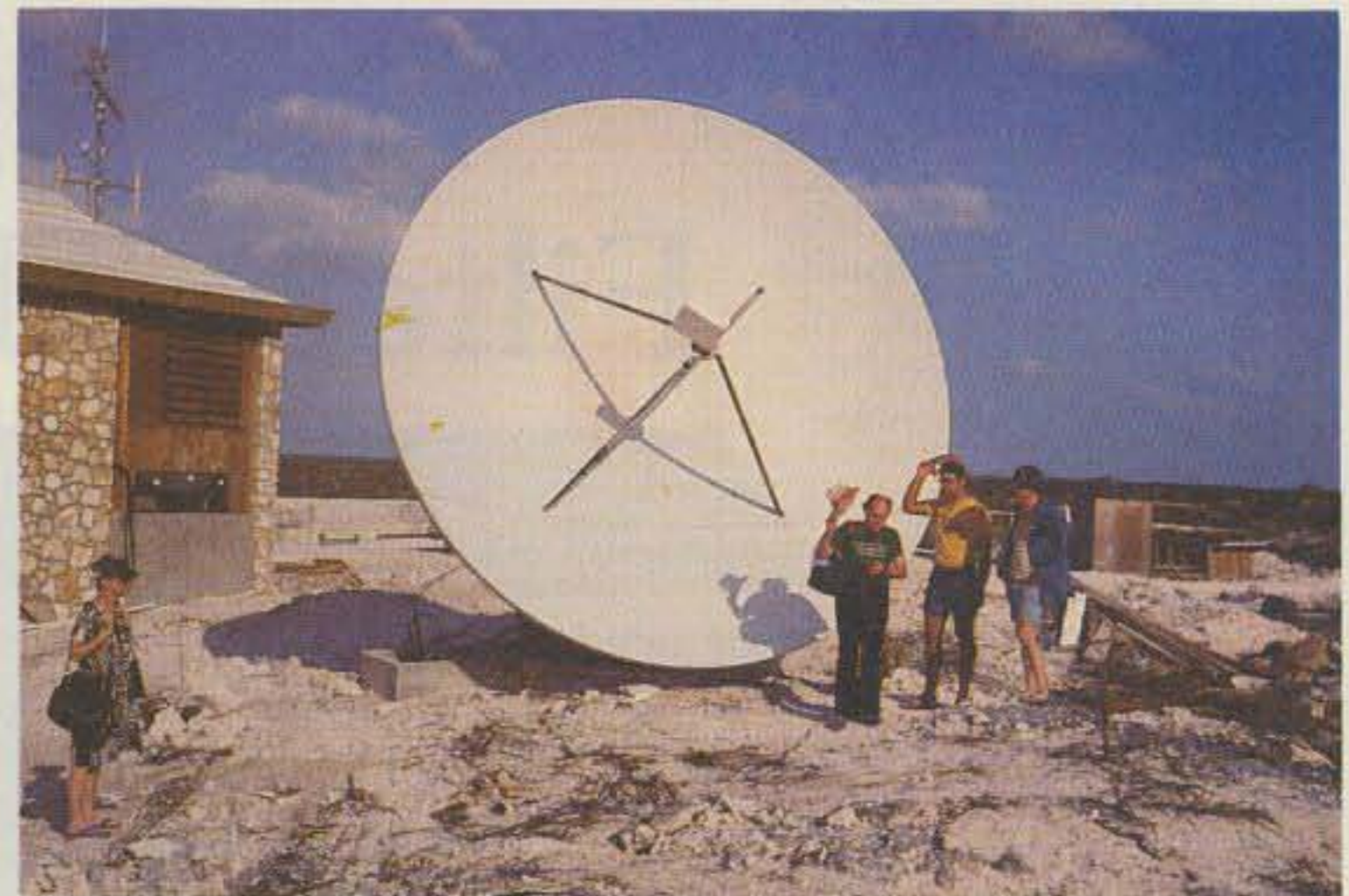
This 20' dish is outside the new WIV television studios. Yes, I know they can't use a "W" prefix in Turks and Caicos. Their answer: "Who says so?" We arrived on a very unusual day . . . when the sun was exactly behind the satellite, thus creating a good deal of sun noise on the signal. Notice shadow of the LNA (low-noise amplifier) in the exact center of the dish. It happens about once a year. That's me, Coop, and Chuck, with Sherry carrying my camera bags.
