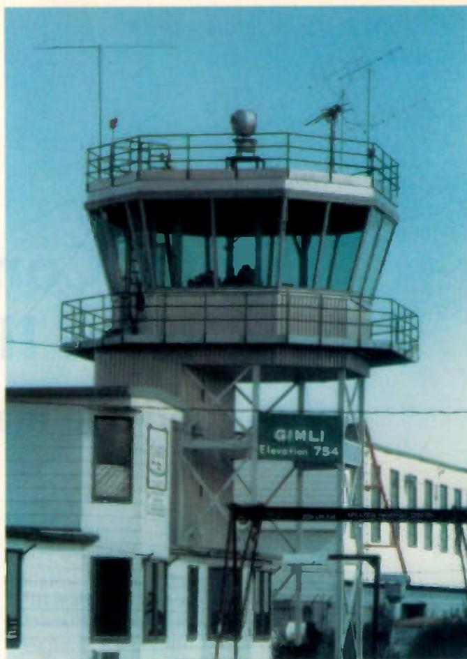
The Gimli control tower. The 4 × 6-element yagi for 2 meters is seen to the right and the 432-MHz beam can be seen to the left.
