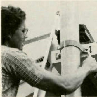
Mounting the House Bracket
