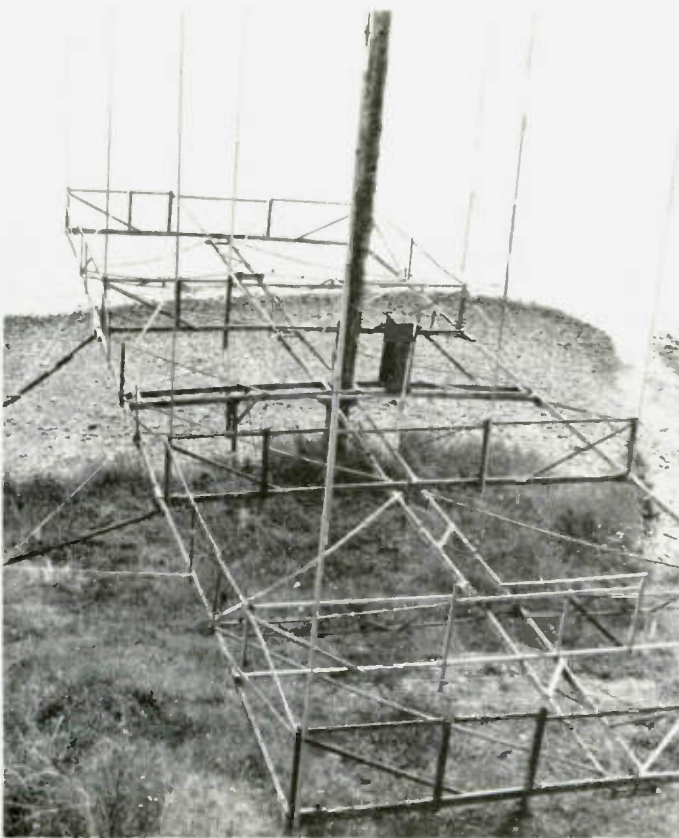
This photo was taken from the roof of Tom's home. The camera is facing east, with the boom facing south. The box contains the tuning unit to protect it from the weather. The ten nylon lines supporting the boom are shown in this photo.
