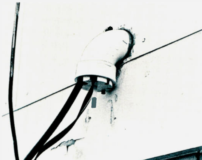
Outside view of the 90° elbow installed with an antenna cable already routed through.
