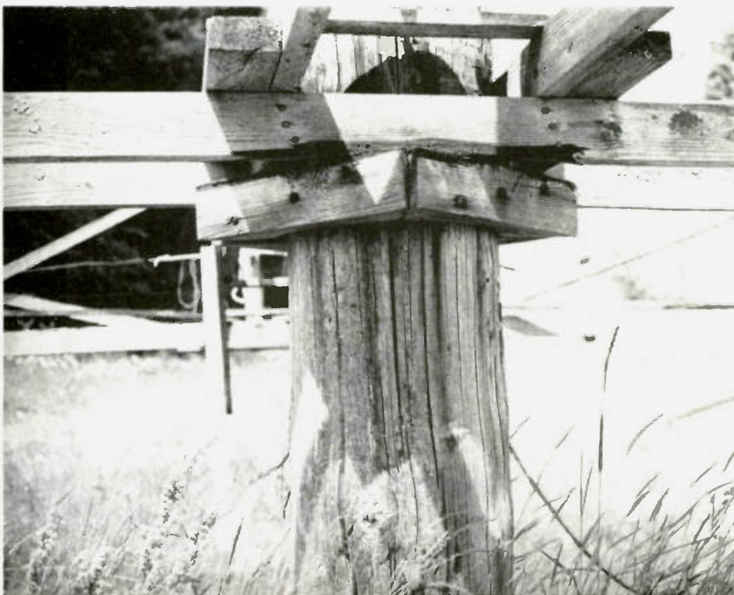
The bearing is kept well greased and supports the entire array with the aid of the ten nylon lines.
