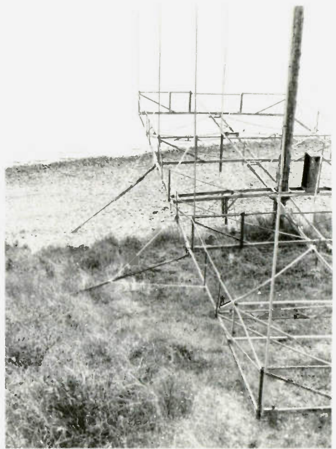
Close-up showing 12' 2 x 3s, which prevent rotation by the wind and which are used to turn the boom by hand.
