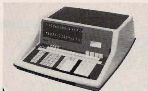
The Wang 700A -- a powerful desk top calculator with 8,192 bits of memory organized as 120 storage registers. Programs for the calculator are stored on magnetic tape cassettes.
