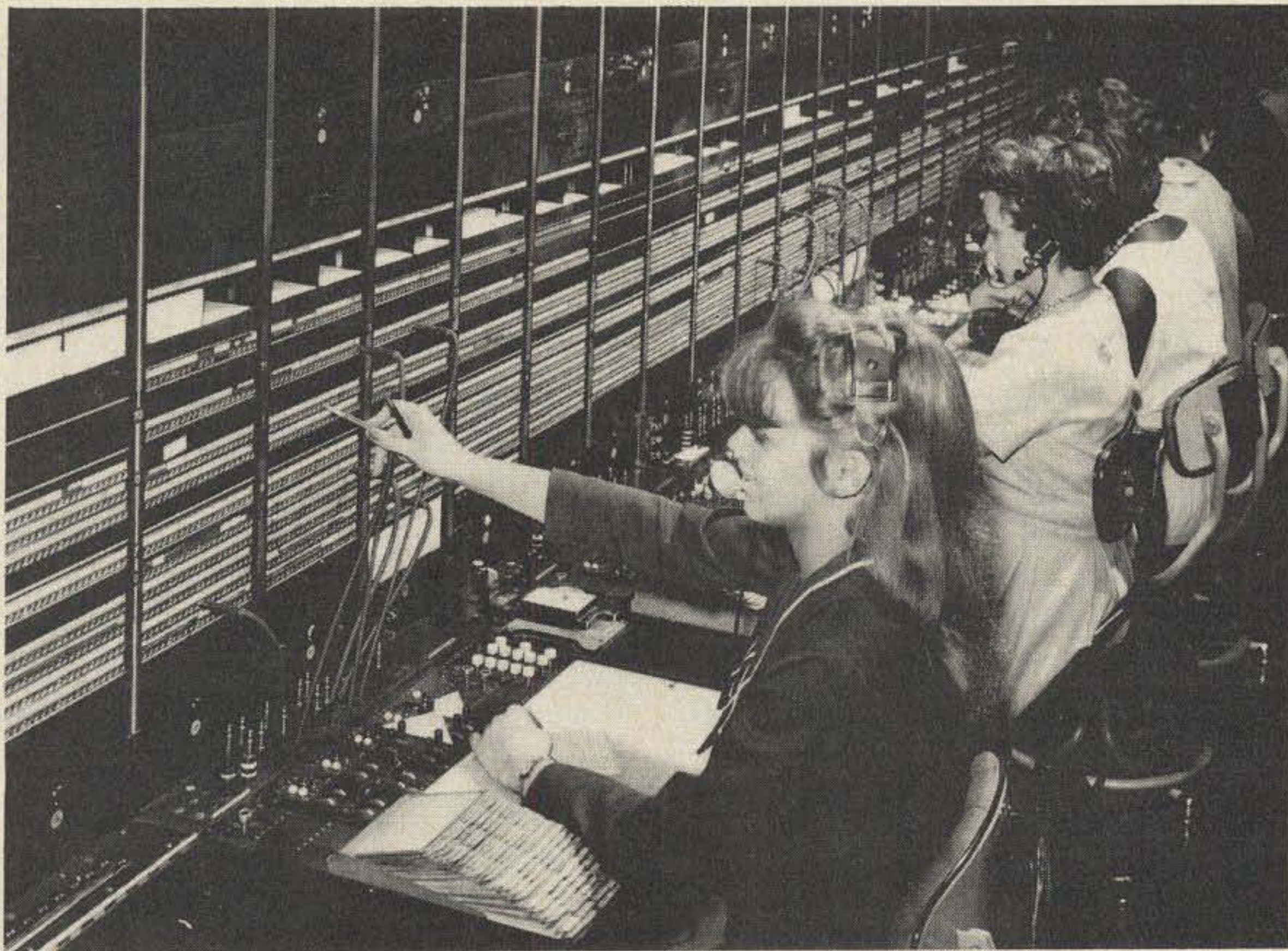
Fig. 1. View of long distance telephone switchboard operations. Pacific Telephone Co. photo.
