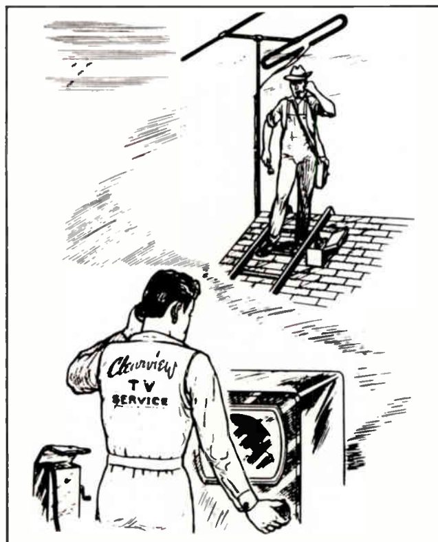
Fig. 12. Two-Way Sound-Powered Telephones are useful in Antenna Installation Work.
