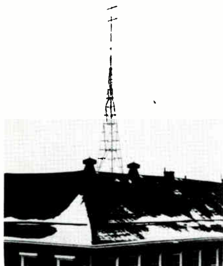
In fringe areas, for good reception, the height of the antenna is important due to line-of-sight transmission characteristics. Shown is a 40 ft. tower and mast designed for roof installation.
