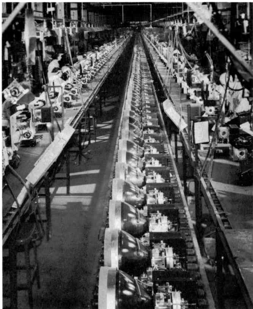
Television chassis come off this assembly line at the rate of one-a-minute. Courtesy Crosley Division, Avco Mfg. Corp.
