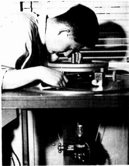
Aligning the shadow mask with the phosphor screen requires precision.
