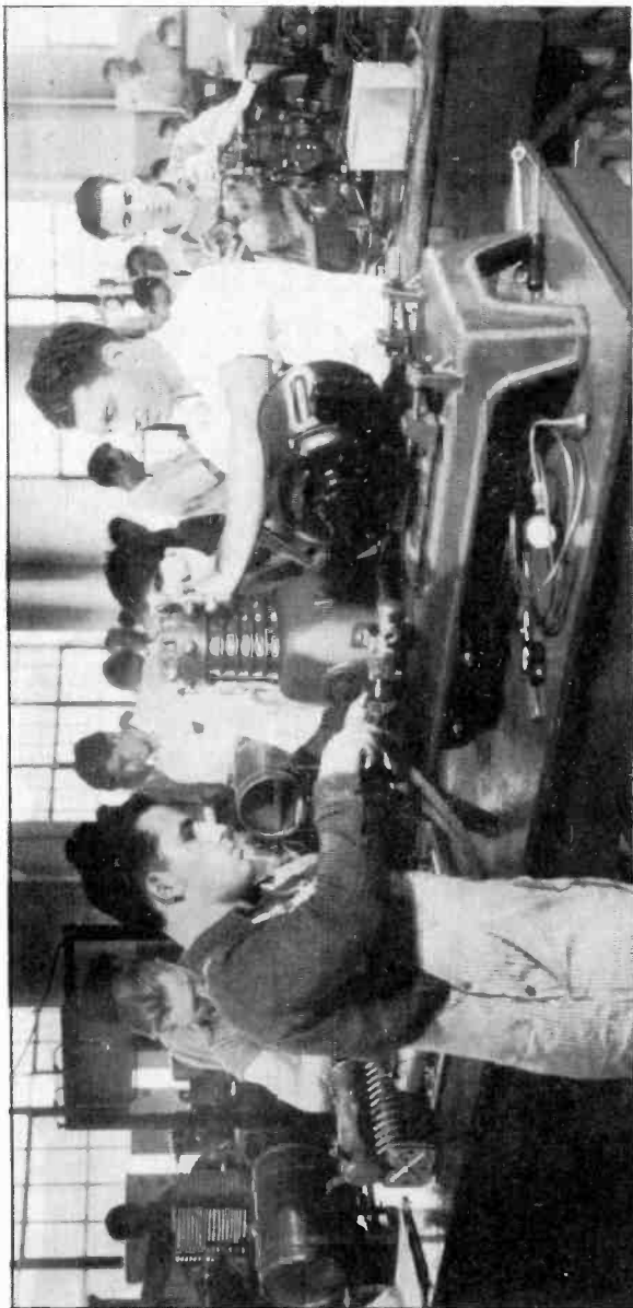
Refrigeration servicing offers great opportunity for the trained man. This view shows a modern compressor being adjusted. Thousands of these compressors are used in both commercial and household refrigeration units.
