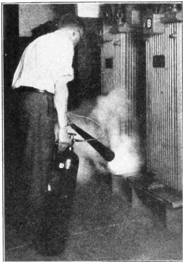
Fig. 12. This photo shows the use of a modern gas type fire extinguisher for fire protection in electric plants.
