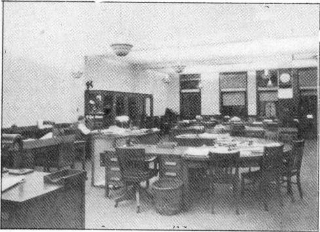
Fig. 4. This office is lighted with indirect units which are ideal for avoiding all glare and shadow effects. (Photo Courtesy Light Magazine).
