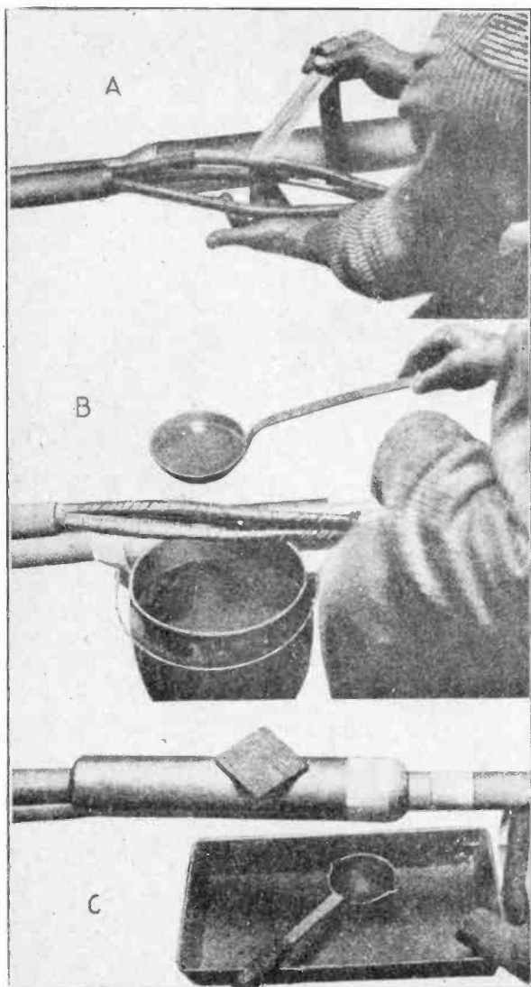
Fig. 13. This view shows several of the important steps in splicing lead covered cables.
