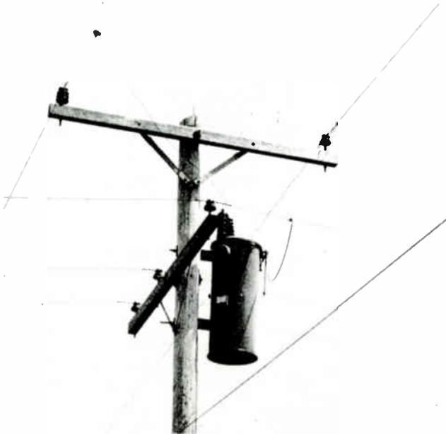
Fig. 25 This transformer reduces the power transmission voltage down to 115 and 230 volts for use in nearby homes.
