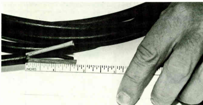
Fig. 29 Strip off 1-1/2 to 2 inches of the outer cover, exposing the three insulated conductors. The length of exposed insulated conductor depends on the type of receptacle you have. For the receptacle shown in the photograph, 1-3/4 inches was the proper length. Take care not to nick the insulation on the conductors. If you nick the insulation, just clip off that section and strip off some additional outer cover.
