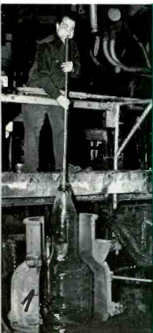
Facing Page —In the manufacture of plate glass, molten glass from the furnace flows over a lip into the forming rolls shown here. A continuous ribbon of glass about 11 feet wide is formed. (photo courtesy Pittsburgh Plate Glass Company)
