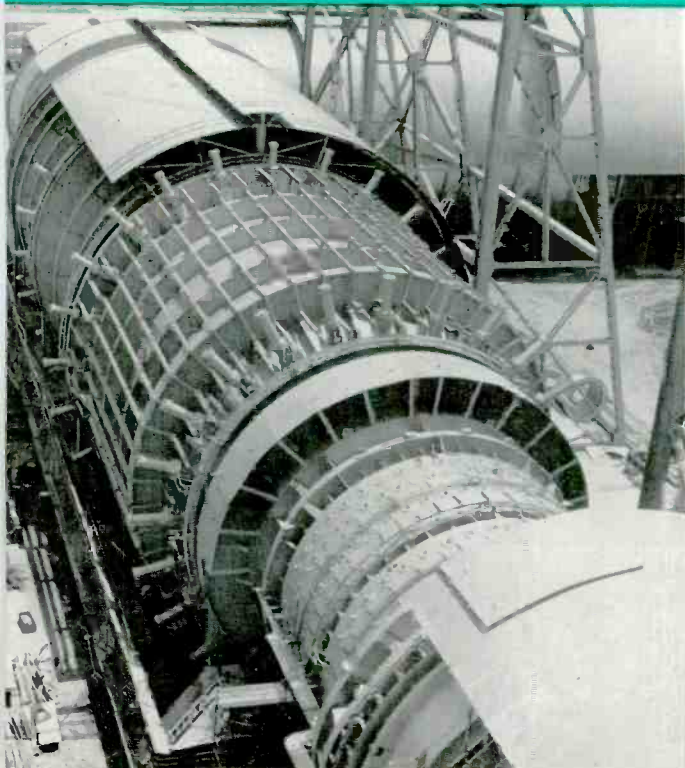
This is a portion of the giant 247-foot long supersonic compressor unit. Four compressors, with a total of 21 separate stages, comprise this entire rotating mass.
