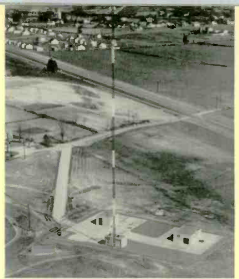
A booster station operated by supervisory control over microwave. From left to right are the outdoor substation, control building, microwave building and tower, and pump building.
