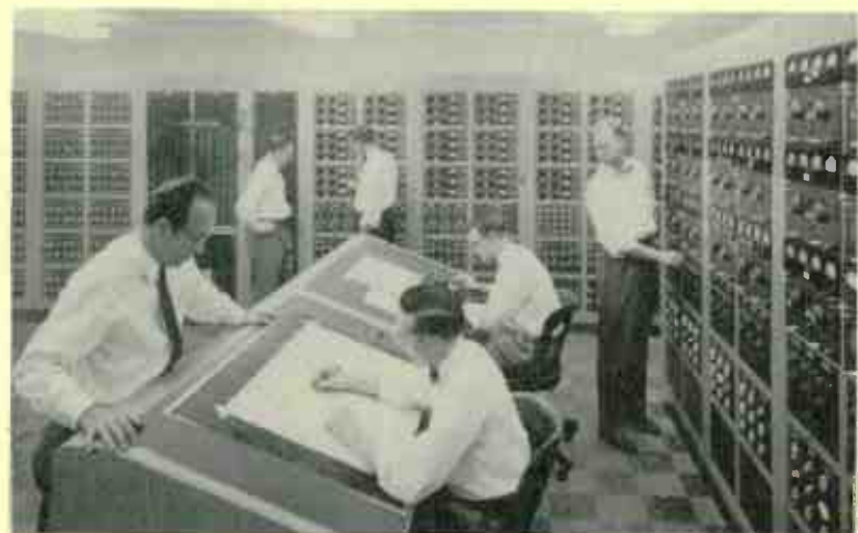
A new a-c calculator, at the Westinghouse East Pittsburgh plant, is designed to accommodate the largest interconnected systems and power pools in existence. Background is a section of the board.
