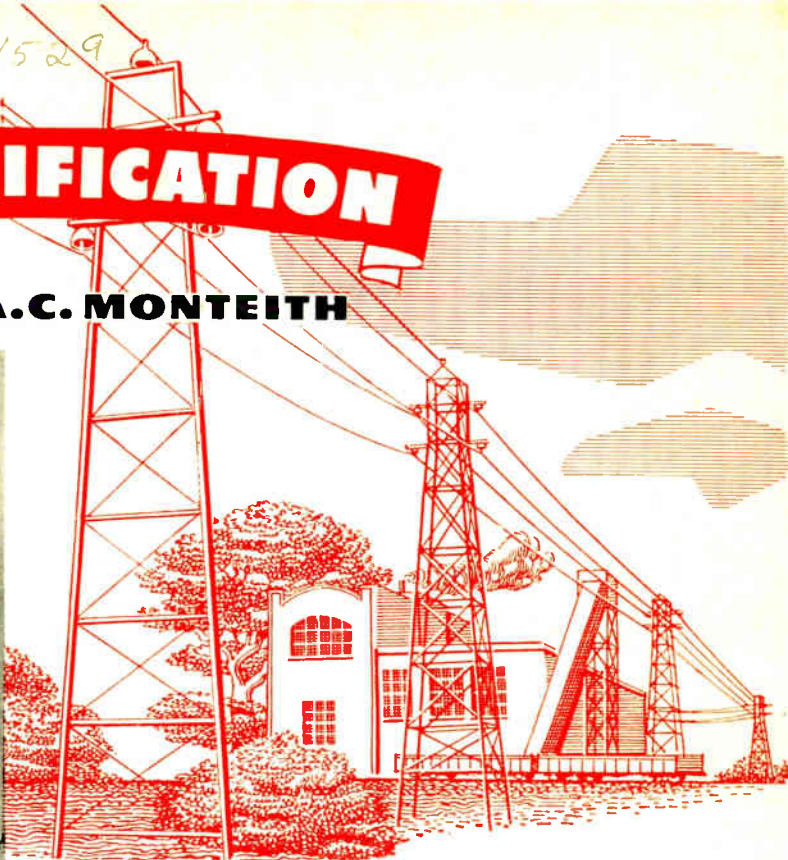
Station and transmission line of 1911
