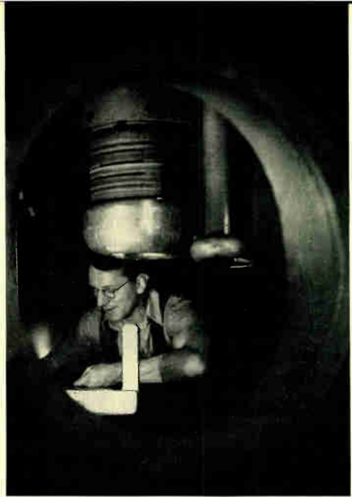
Fig. 9—View through the manhole of a 230-kv breaker having a special 1250-ohm voltage-damping resistor.
