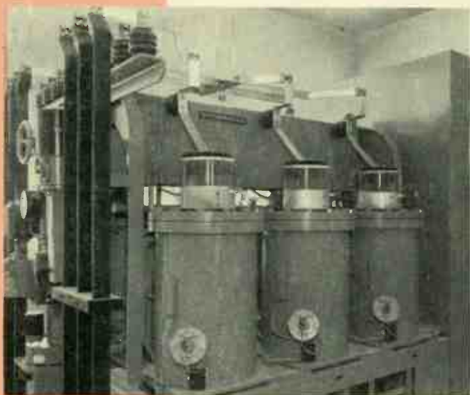
Pumped ignitrons have taken the step to higher voltage. This 3000-kw, 3000-volt rectifier is supplying power to mining locomotives in Utah. The rectifier, with special grid and extra heavy construction, has been able to operate very successfully at this high voltage even with the sudden, large load swings of mining service.
