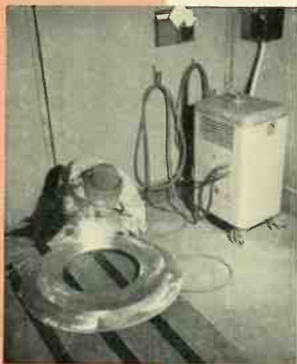
Pumped ignitrons have taken the step to higher voltage. This 3000-kw, 3000-volt rectifier is supplying power to mining locomotives in Utah. The rectifier, with special grid and extra heavy construction, has been able to operate very successfully at this high voltage even with the sudden, large load swings of mining service.
