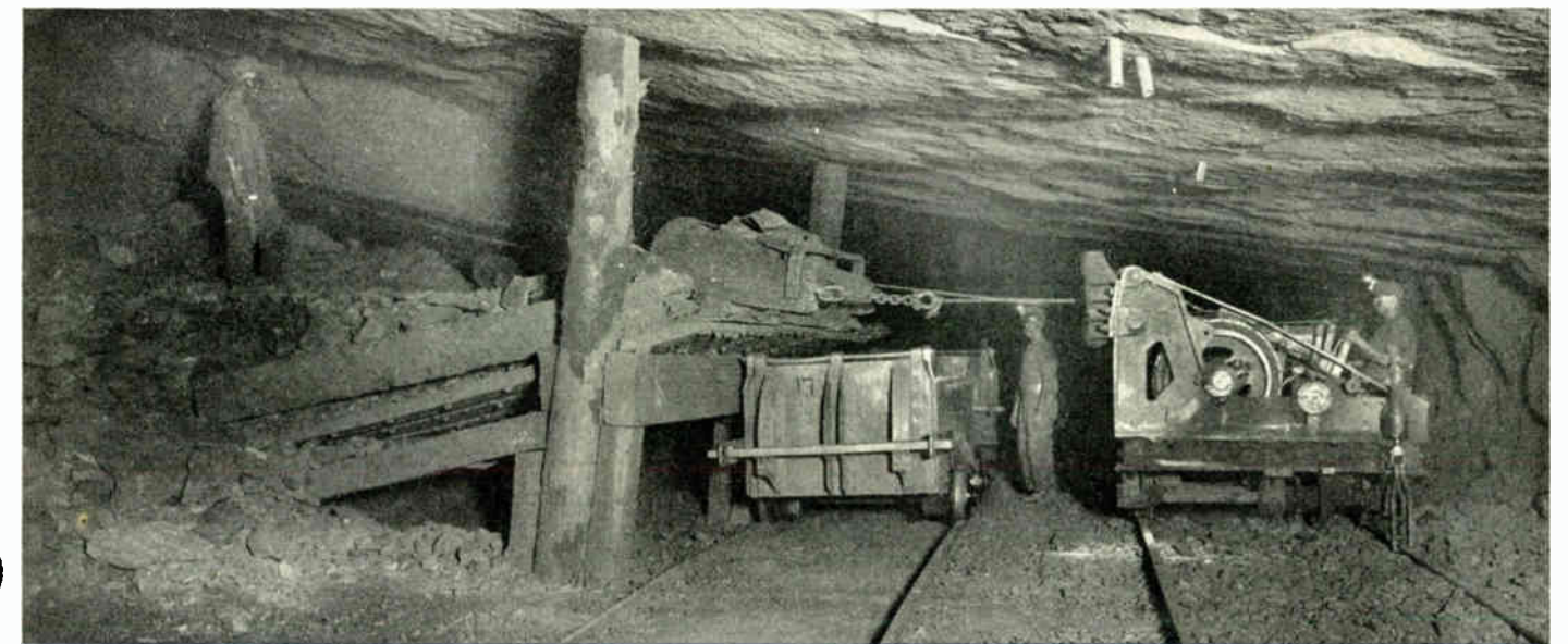
Iron ore starts on its journey from mine face to blast furnace in this mine of the Tennessee Coal and Iron Company near Birmingham.
