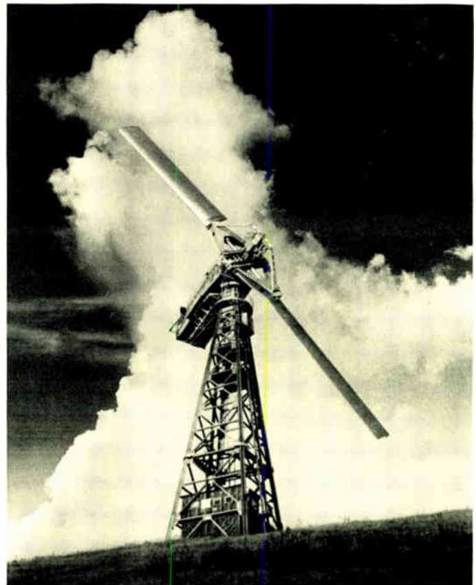
... The windmills of Holland and the American farm-yard have captured much useful power from the winds, but it is insignificant compared to our needs. On Grandpa's Knob on a Vermont mountain top is this wind-driven power plant, delivering at full load 1000 kw. (Photo courtesy S. Morgan Smith Company.)
