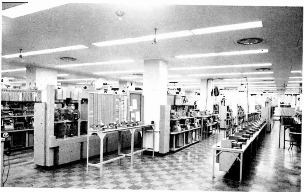
Figure 3. Mastic tile flooring, flush fluorescent ceiling lights and ceiling ventilating outlets—Philadelphia
