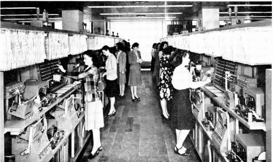
Routing lists are displayed above operating positions in Philadelphia switching center
