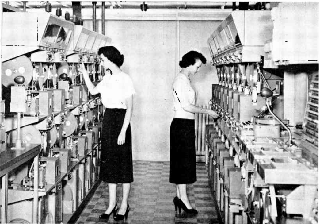
Figure 13. Sending racks—Portland switching center
