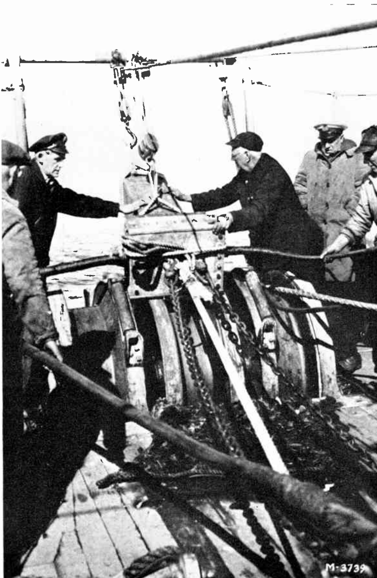
Figure 15. Repeater passing over bow sheaves
