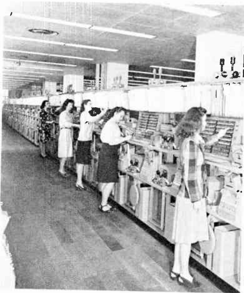
Figure 2. Flush fluorescent ceiling lights, cork flooring and ceiling ventilating outlets—Philadelphia switching aisle
