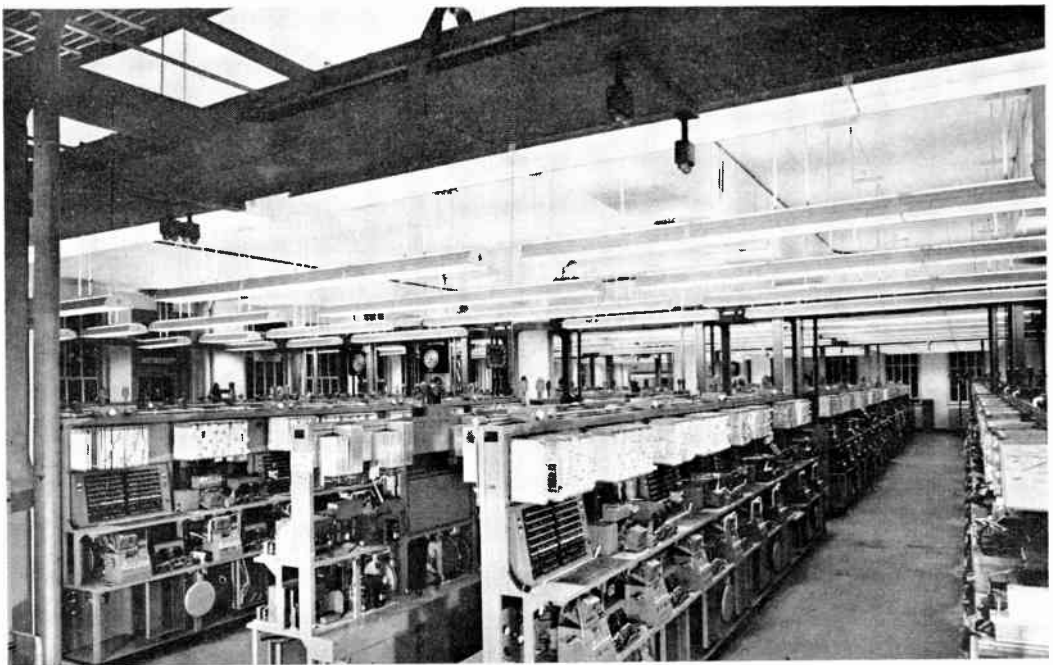
Figure 1. Cincinnati reperforator switching center with fluorescent lighting suspended below ceiling
