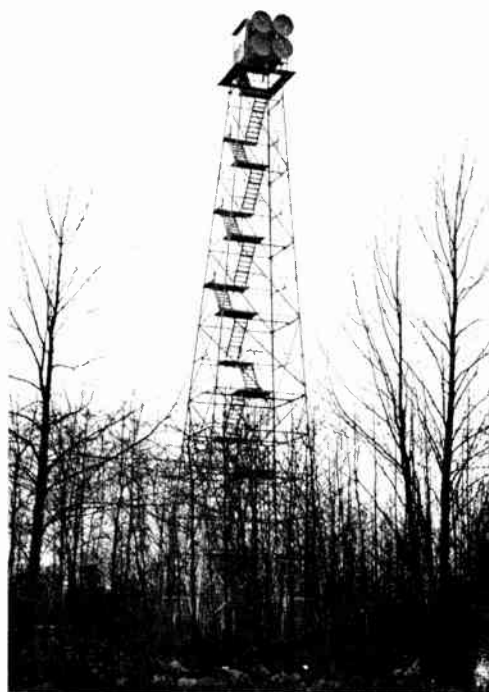
Figure 1. Neshanic propagation tower
