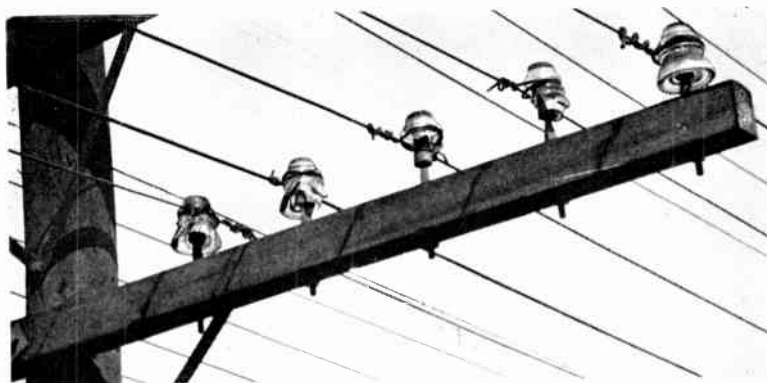
Figure 1. Illustrating mischievous damage to glass insulators
