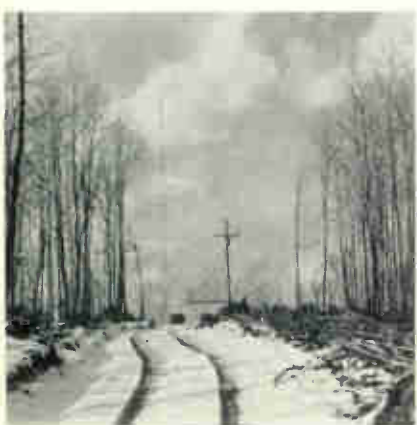
Figure 3. The KG2XDU tower and station building.
