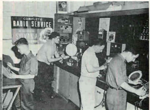
Above: At work at the busy service bench is Gordon Stanys, on television; John Geriah, on a home receiver; Angelo Pellicciari, auto radio; and Nicholas Amenti, checking tubes on a Sylvania Tube Tester. Sylvania Tubes are used as replacements in the sets repaired in the Stolfi shop.
