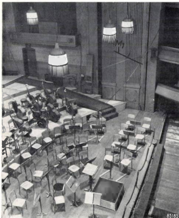
Fig. 5. The stage in the "Gebouw voor Kunsten en Wetenschappen" in The Hague. M_1 is the line microphone (rod with ten condenser microphones). (Other microphones visible in the photograph were for broadcasting and had nothing to do with stereo reverberation.)
