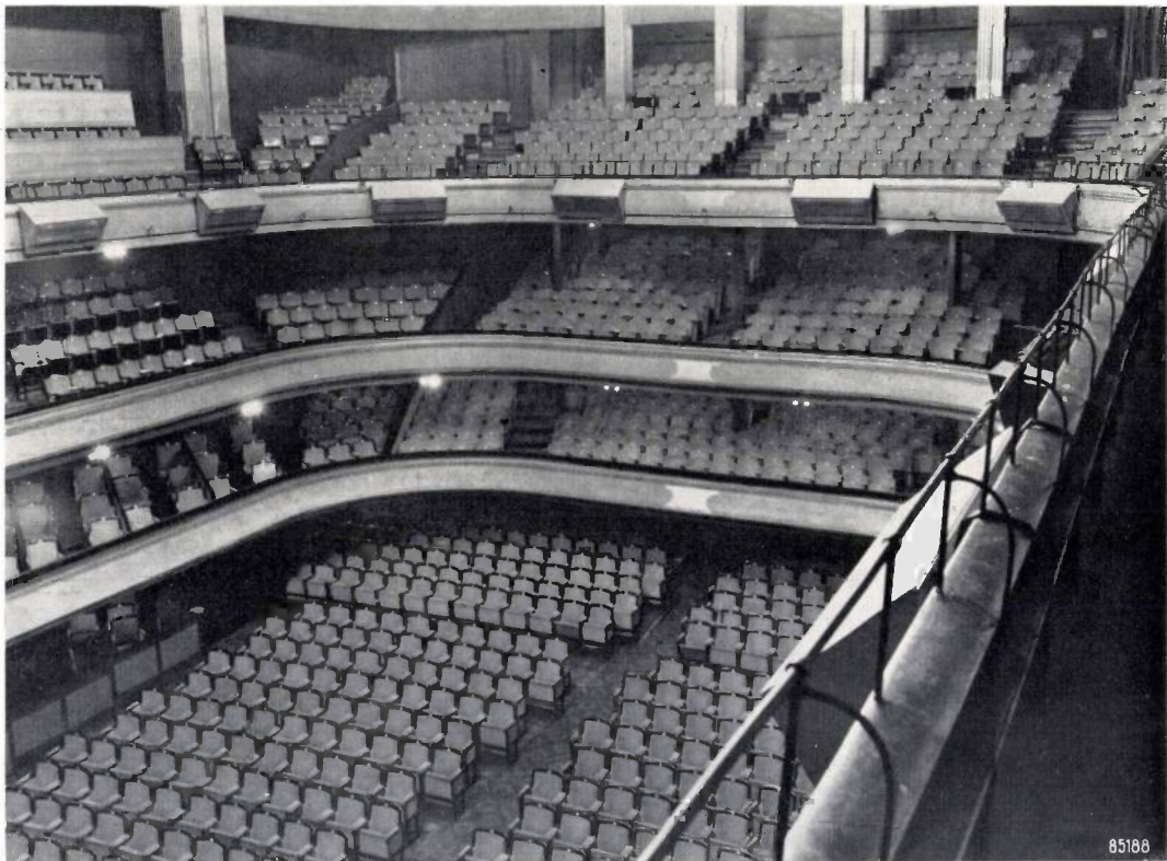
Fig. 8. In the "Gebouw voor Kunsten en Wetenschappen" the loudspeakers are mounted along the edge of the upper balcony and (not visible in the photograph) under the balconies.
