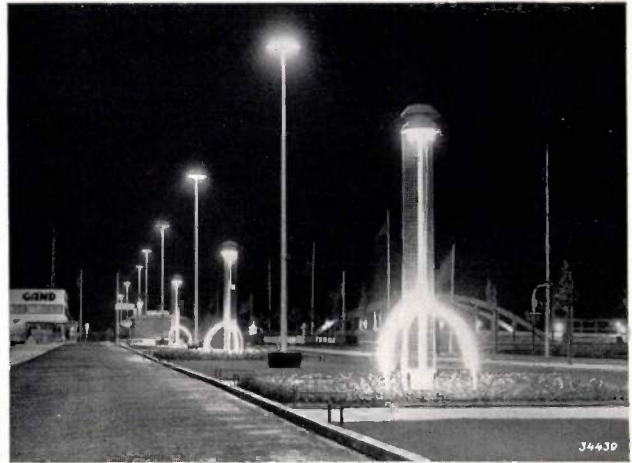
Fig. 2. Between the stadards for the boulevard lighting, stand the light ornaments for illuminating the flower beds. They are five m high and bear a loud speaker and three milkglass globes each with a 150 dlm lamp. The strips of netting are lighted with "Cornalux" lamps.
