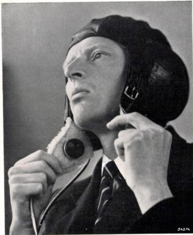
Fig. 9. The laryngophone can easily be fitted into an aviator's helmet.
