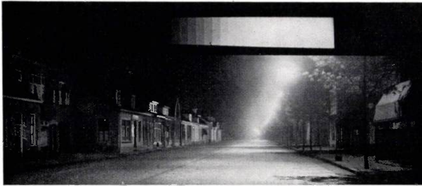
Fig. 11. Road provided with ZE 30 fittings in which are mercury lamps 125 W MB/V (5000 lm). Height of suspension of the light sources 9 m, spacing 34 m. All the sources are on the same side of the street above the curb. Width of street curb to curb 12 m. Dry road surface. Above is a series of density standards for the determination of the brightness of every point on the road surface; see the article cited in footnote 1 ).
