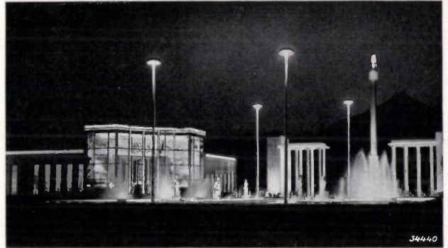
Fig. 4. The great square behind the entrance is illuminated by four 20 m high standards of construction similar to that in fig. 1. The cap on each standard in this case however contains three mercury lamps, type NO 2000, and three 1500 watt electric lamps, which together give a light flux of 13 500 dlm.
