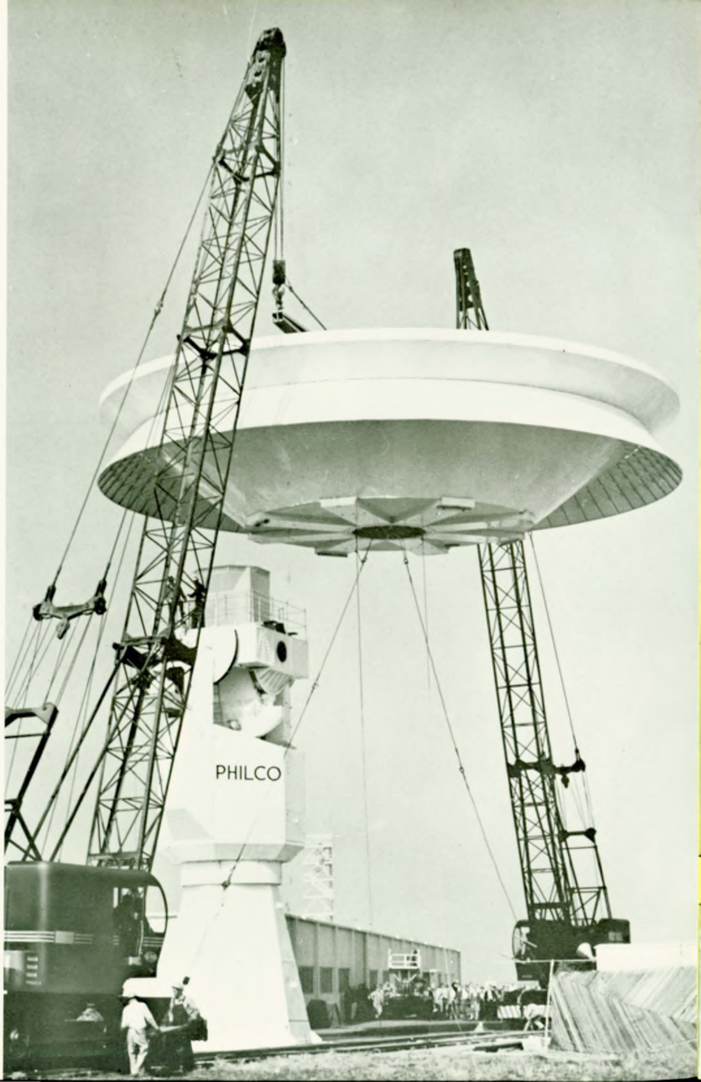
Satellite tracking antenna designed and constructed by Philco
