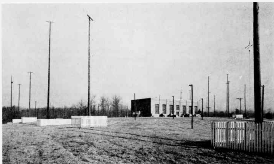
Figure 15. Exterior of NBS Radio Broadcasting Station WWV, Beltsville, Maryland. From this station, standard radio frequencies of 2.5, 5, 10, 15, 20, and 25 mc. are transmitted continuously with accuracies of two parts in 100 million. Two standard audio frequencies, 600 and 440 cycles, are broadcast on all radio frequencies. Telephone poles support the antenna system, from which signals are transmitted to all parts of the world.
