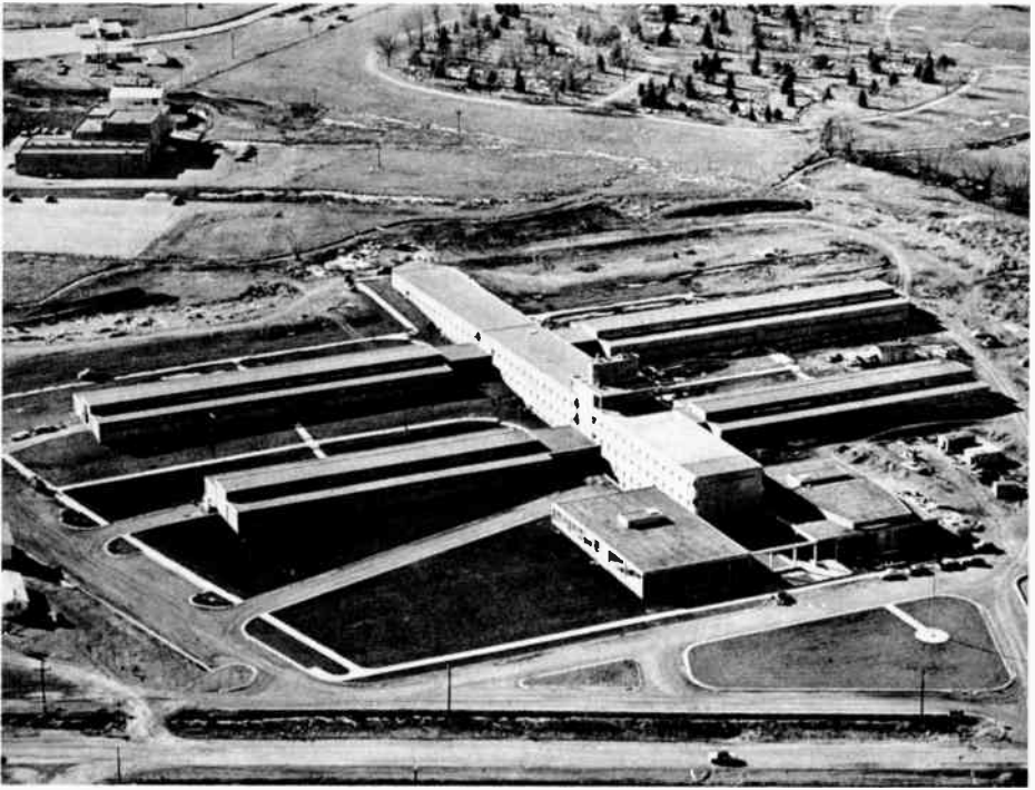
Figure 1. Air View of the National Bureau of Standards Multimillion Dollar Research Center in Boulder, Colorado. This structure will house the Bureau's Central Radio Propagation Laboratory. The design of the building features a central spine, with one-story wings extending perpendicularly from it on either side. The structure takes advantage of the sloping terrain that rises from a state highway toward the Flatirons to the west. The buildings in the background, also part of the research center, are portions of the NBS-AEC Cryogenics Engineering Laboratory.
