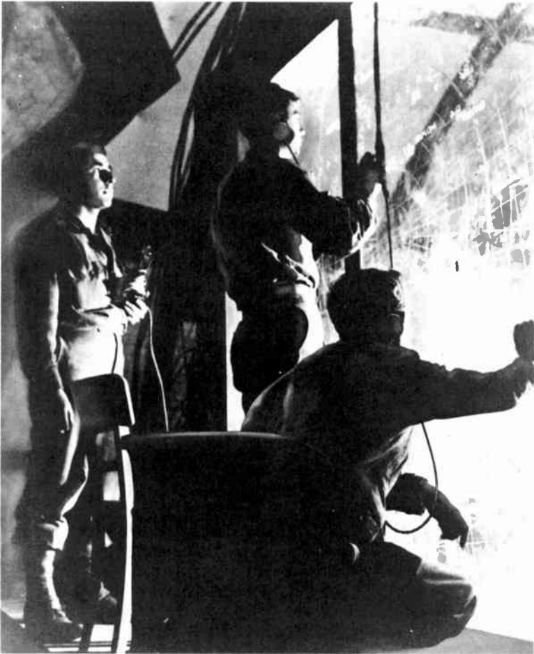
Figure 6. Plotters Behind Vertical Plotting Board, Tracking Aircraft (Writing is done backward so as to be correct when viewed from front.)
