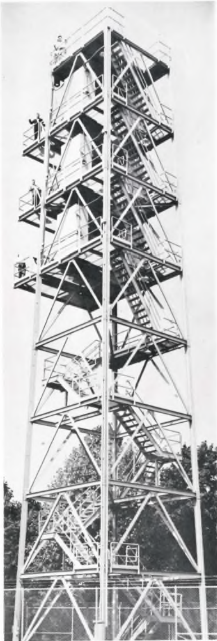
Four Philco research staff members stand watch on levels of the Division's microwave antenna tower in Blue Bell, Pa. The 100-ft. structure's four levels are designed to accommodate transmitting equipment for simultaneous transmission of narrow microwave beams to the new Philco Research Center located eight-tenths of a mile to the southeast. Study and evaluation of experimental radar antennas is an important activity of the Microwave Techniques Section of the division.
