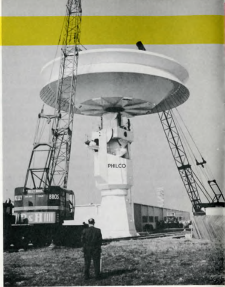
Sixty-foot reflector for world's largest three-axis antenna resembles giant bird bath as it is mounted atop 50-foot pedestal at Philco's Western Development Laboratories, Palo Alto, California. Destined for a remote satellite tracking station, the antenna is largest in world to employ tri-axial mounting—movement in three directions much like a man's wrist and forearm. Antenna will provide hemispheric coverage of telemetered information and data from satellites and missiles during any phase of flight.
