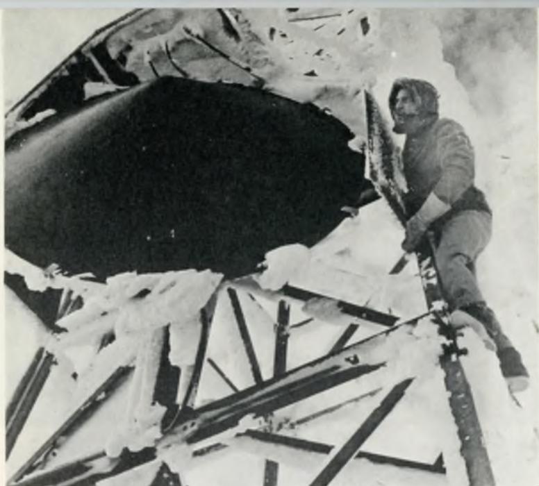
This is not Alaska, but a Philco Microwave repeater antenna on Mount Spokane in Washington State. An Engineer of the Communications Systems Division checks the operation of the Philco Thermo-Microdome covering that keeps the snow and ice from the dish antenna.
