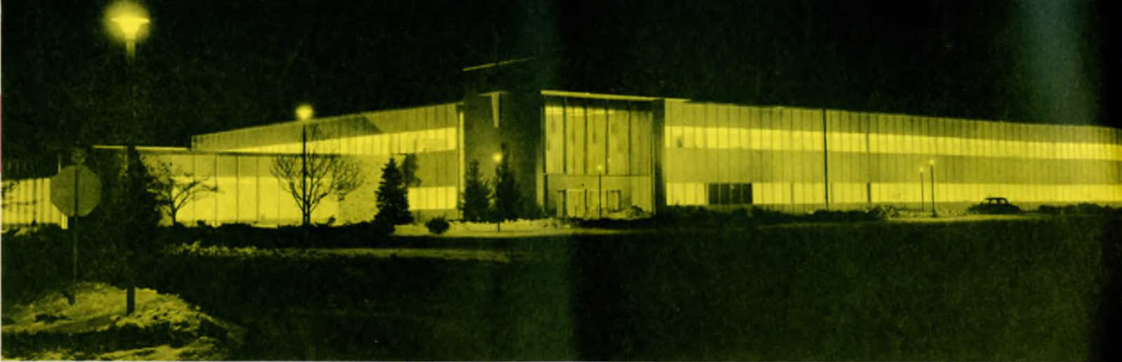
A night view of Philco's new computer center at Willow Grove. This ultra-modern plant has over 200,000 square feet of floor space. The national sales offices and research, engineering and manufacturing
