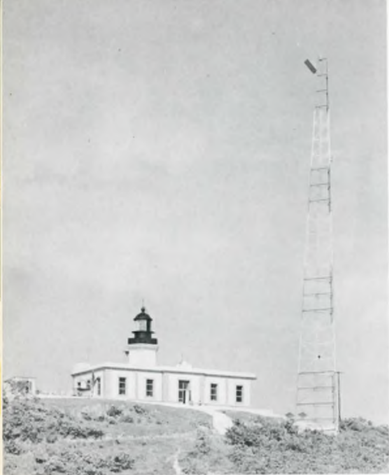
▶ This lonely lighthouse, located on the Northern Coast of Puerto Rico, was joined by a Philco Microwave repeater, part of the system that provides telephone and teletypewriter communication between Ramey Air Force Base and Fort Buchanan. A similar system will be installed near Fort Allen, Puerto Rico, by the Installation Engineers of the Communications Systems Department.
