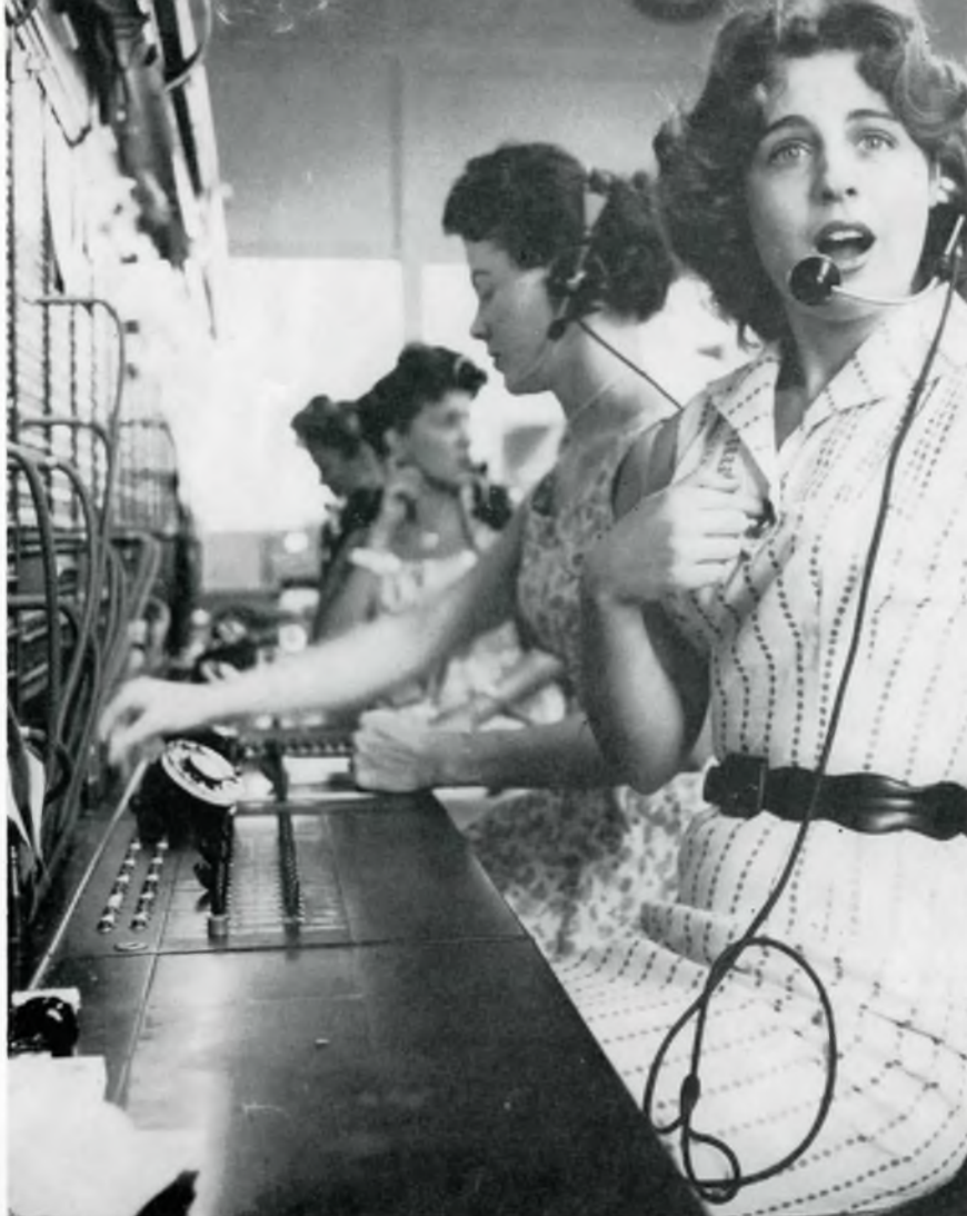
Joan Finn, Plant 50 Telephone Room, asks a question answered below.
