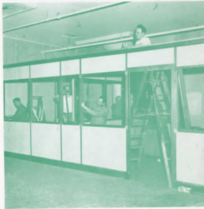
PARTITIONS FOR NEW OFFICES to be located on the first floor of Plant 2 are installed by Richard Arwood, Harry Wagner, Louis Curran, Charles Owens and Louis Hebson.
