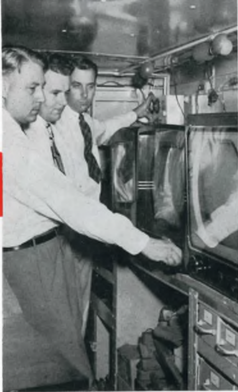
3. With receivers OK under these tests, the mobile laboratories take over and try the receivers in the various troublesome signal areas.
