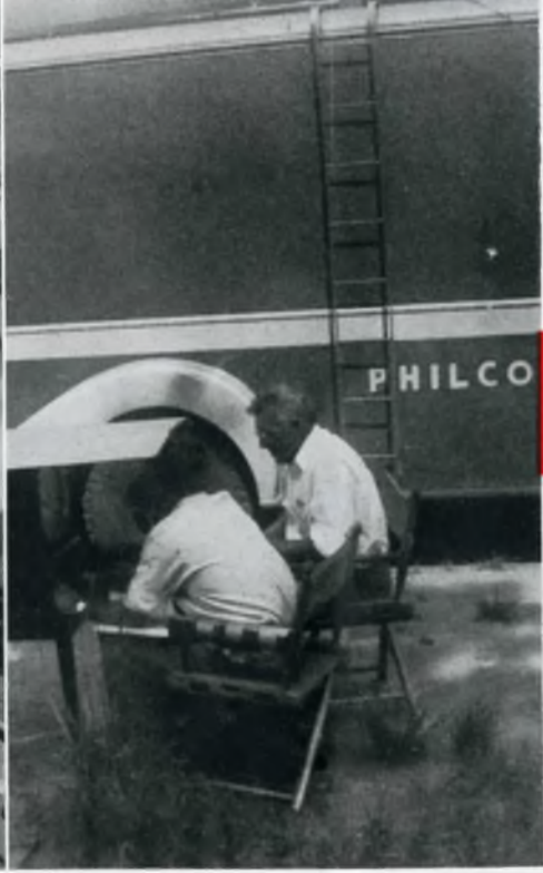
3. With receivers OK under these tests, the mobile laboratories take over and try the receivers in the various troublesome signal areas.
