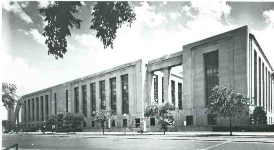
Figure 6 — Headquarters and studios for Voice of America are located in the Department of Health, Education and Welfare Building, 330 Independence Ave., Washington, D.C.
