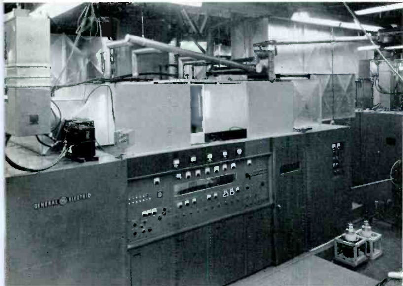
Figure 3 — Front view of the new 250 kW AM transmitter manufactured for the Voice of America by the General Electric Company.
