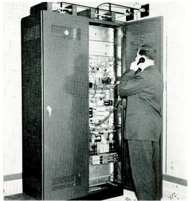
Figure 2 — Portion of microwave relay equipment in New York City.
